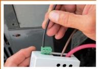
8. Attach the black wire (supplied) to Compressor Common on the NuStart green terminal connector.
