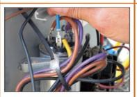
11. Attach the flagged end of the blue wire to the other terminal#2 of the Run Capacitor. Ensure that this terminal on the capacitor also joins to the Start Winding of the compressor.
