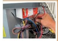
13. Remove the loose wire (from Step 7) from the active input of the contactor and attach the stripped end of the Active wire in its place.
