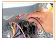
9. Attach the flagged end of the black wire to the Compressor Common on the "T" side of the contactor.
