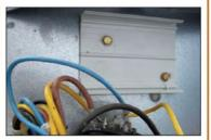
2. Secure the mounting bracket for the NuStart inside the control
