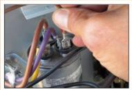
7. Identify the cable connecting the contactor and the Run Cap. Remove this connection to the Run Cap Attach the flagged end of the brown wire to the same terminal of the Run Cap#1.
